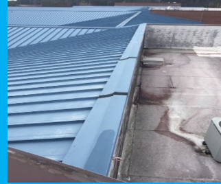
Parapet Metal Cap to be Replaced
