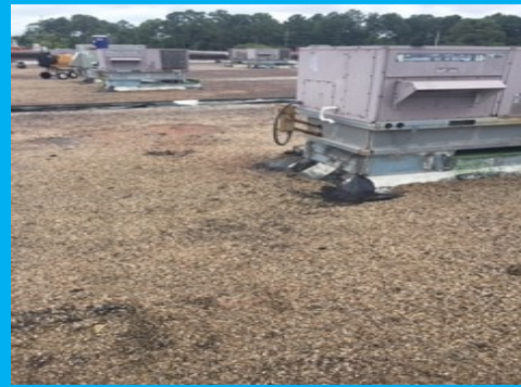
All Flashings around HVAC Curbs Repaired
