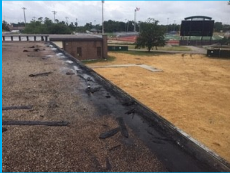
Prep Work for New Gravel Stop
