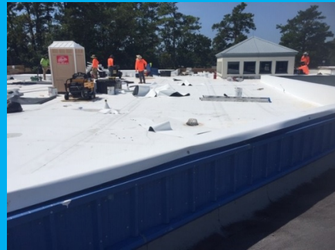
TPO Roof Membrane and Half Sheets
