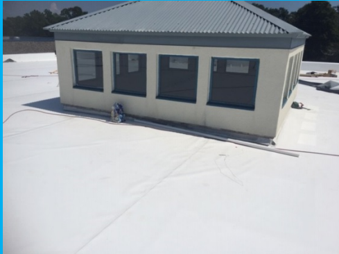
New TPO Roof Around Clerestory
