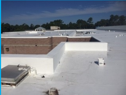
TPO Membrane before Parapet Cap
