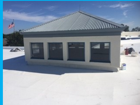
New TPO Flashings around Base of Clerestory
