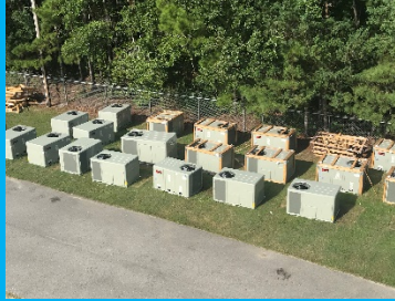
New RTUs (prior to installation)
