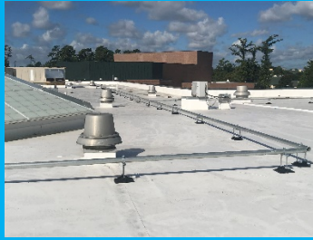
New Galvanized Piping
