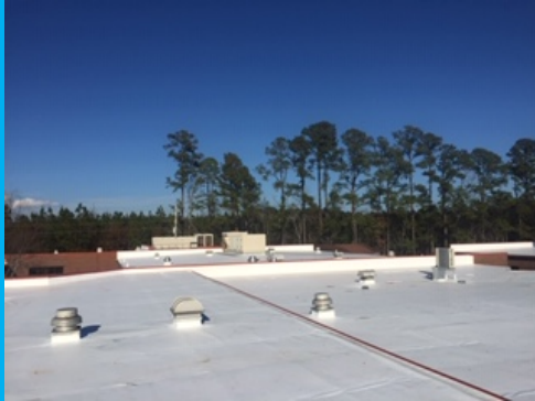
Finished TPO Roof
