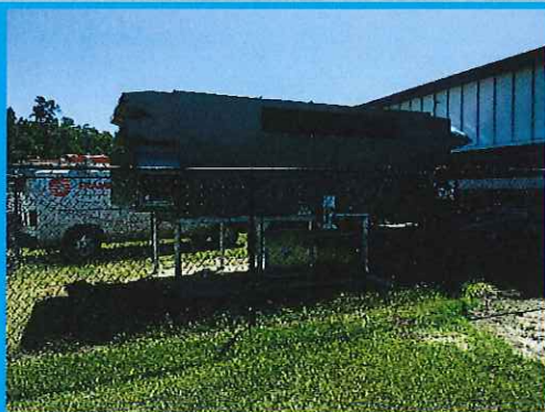
New Outside Air Unit @ Aynor Elem.
