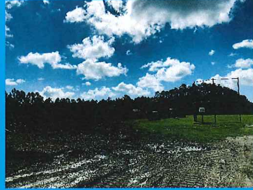
St. James Middle – Bus Lot Cleared & Grubbed
