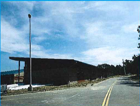
Roof and Exterior Metalwork
