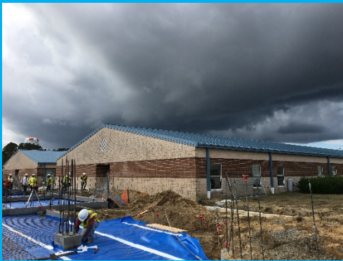
Slab on Grade Construction 80% Done
