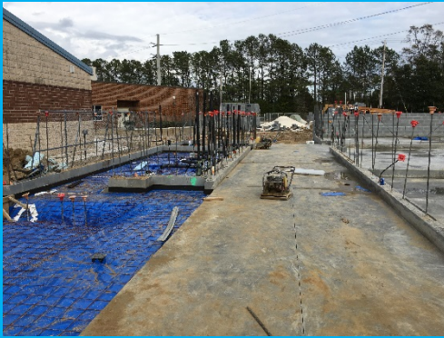
Slab on Grade with Masonry Walls
