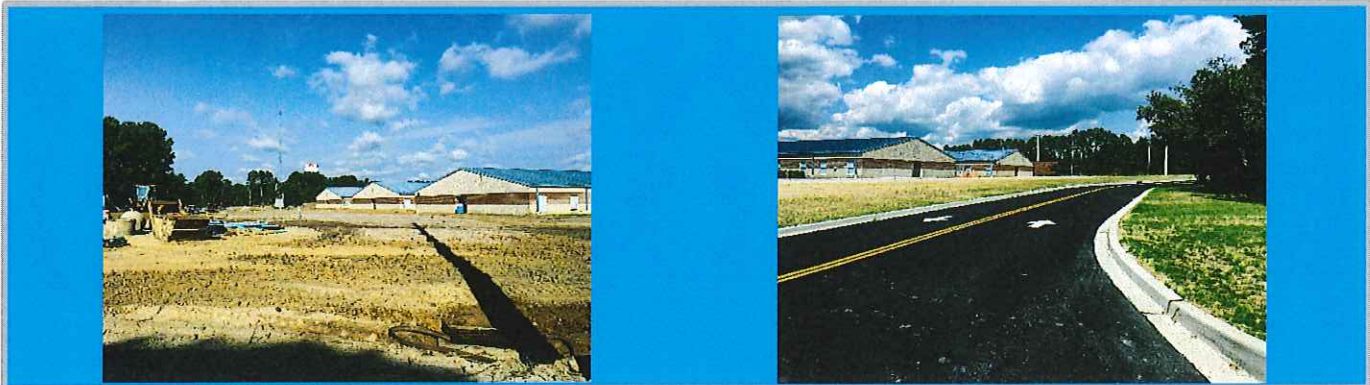
NMBM – Building Pad Graded for Foundation
