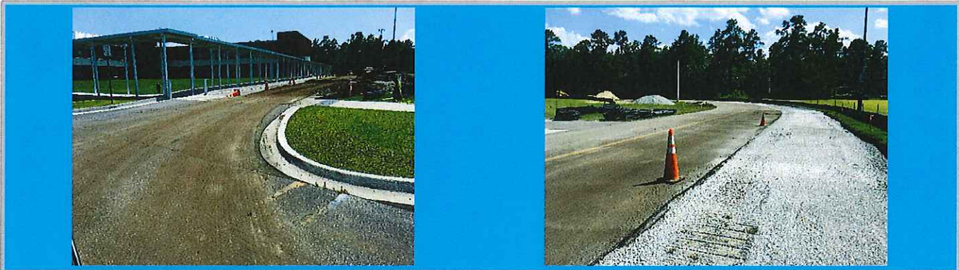
BEFORE - Begin Loop Widening
