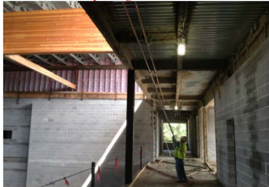
Fireproofing installation
