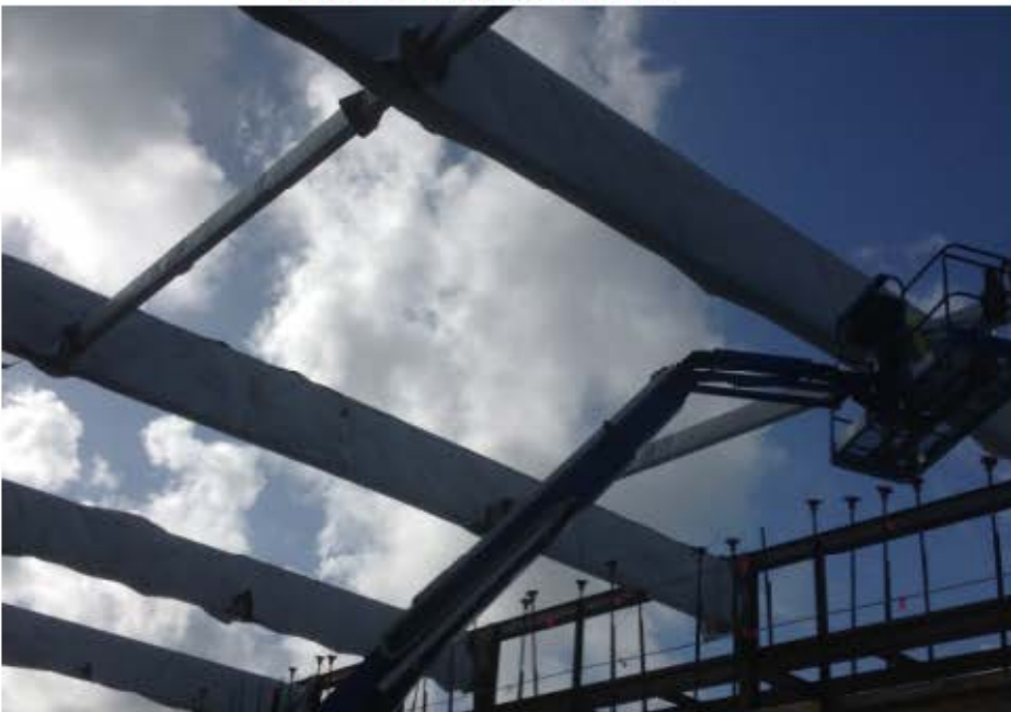
Setting Glulam Beams
