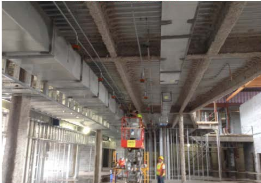
HVAC duct installation
