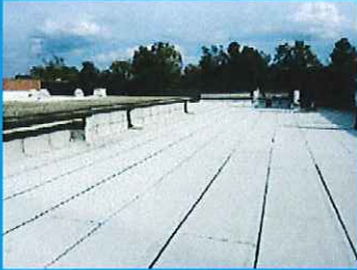
Completed Roof WPMS
